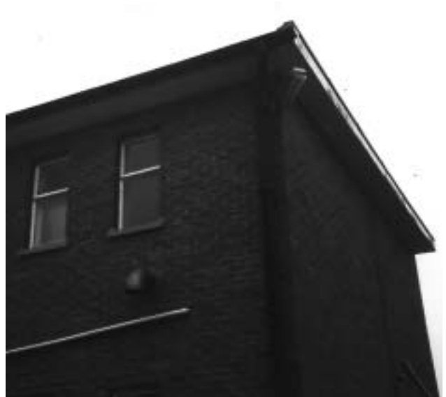
5f Painted AIB soffits.
