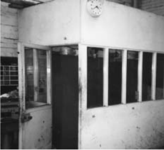
5c Painted AIB partition wall in a factory.
