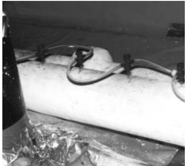
3e Asbestos-lagged pipe with a polymeric encapsulant 'Decadex' finish.
