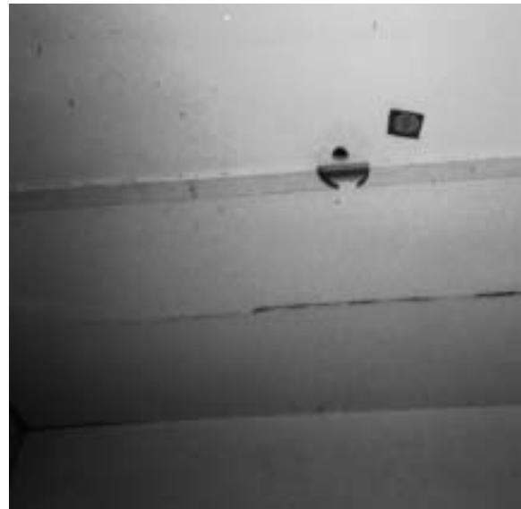
5b Painted AIB on ceiling.
