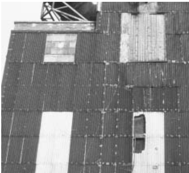
10c Asbestos cement vertical cladding.
