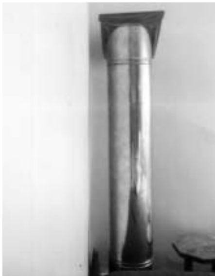
16a Metal-clad asbestos flue pipe.
