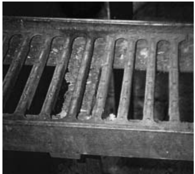
20b Asbestos debris left on a walkway.
