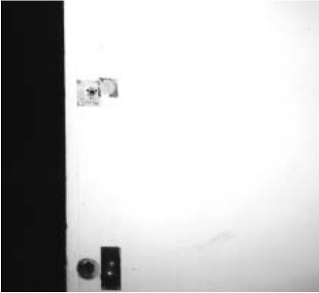
5g Painted AIB facing to a fire door with some damage around the door furniture.
