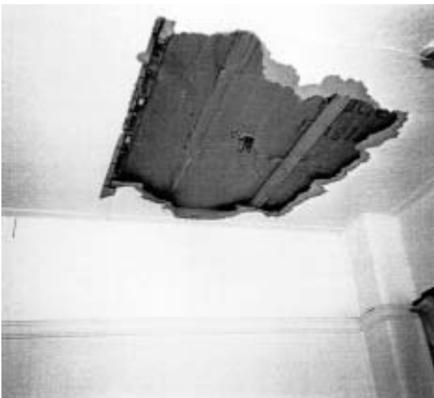
1a Acoustic insulation in a ceiling void with a 'Jiffy bag'-type construction, with paper container punctured for electrical wiring.
