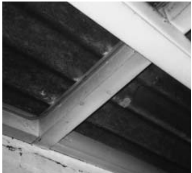
10a Asbestos cement roof (seen from inside).
