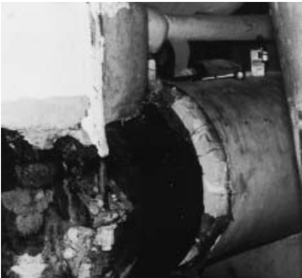
3g High-pressure steam pipes in a power station with a 'Bulldog' finish over 'Caposil' insulation blocks.
