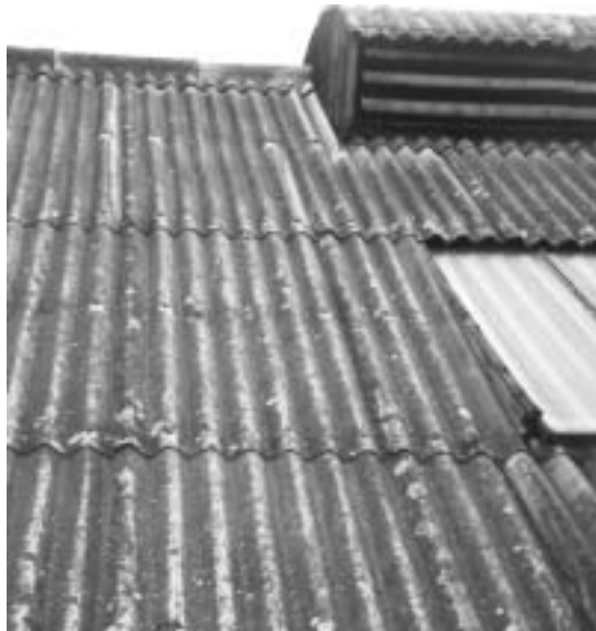
10b Asbestos cement roof (weathered exterior).
